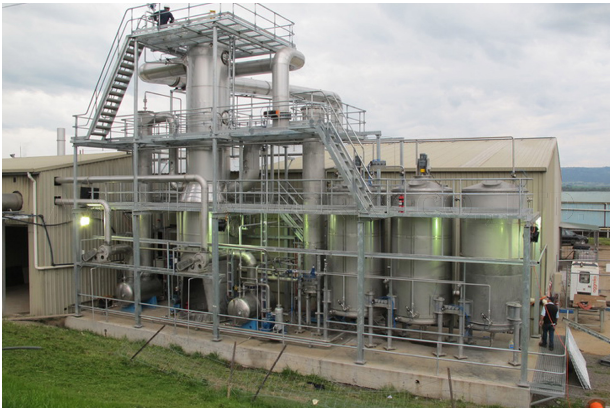
WHE Waste Heat Evaporator with 3 x 10 cum. tanks installed in SCONE NSW AUSTRALIA 2011
