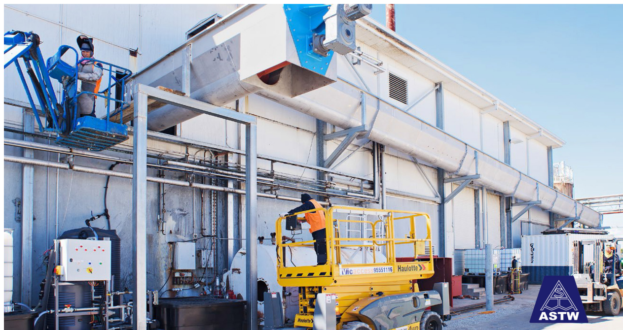
Screw conveyors during installation at abattoir/rendering plant in Australia
