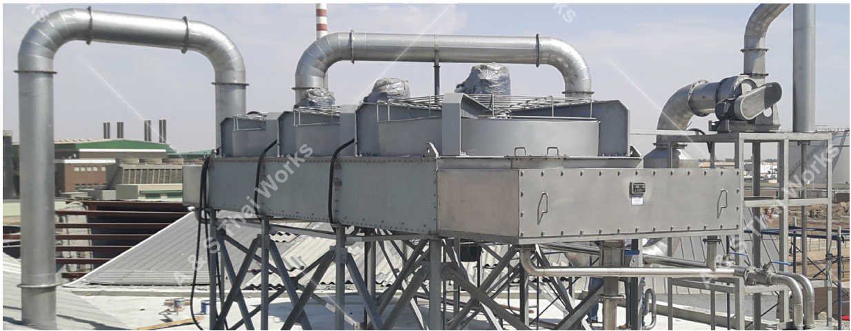
Air-cooled condenser at ASTW fish meal plant in Namibia
