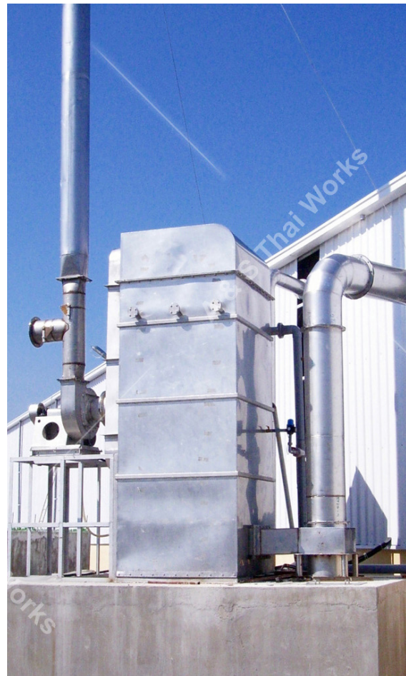
Water scrubber with holding tank at ASTW fish meal plant in Vietnam
